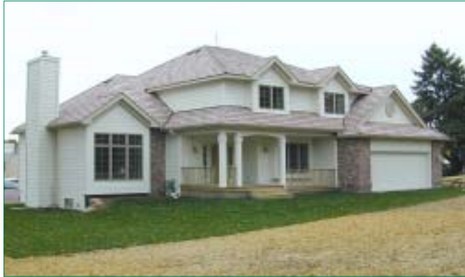
The advanced wood-frame design of FPL's demo house includes energy-saving technology, recycled materials, water-conserving plumbing fixtures, and improved durability.
