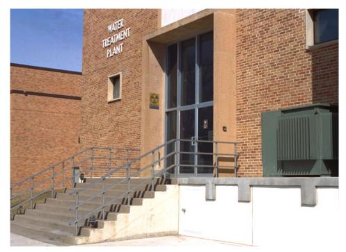
A key electrical transformer (right) has a new home atop this concrete platform, built to keep the equipment high and dry in a future flood.
