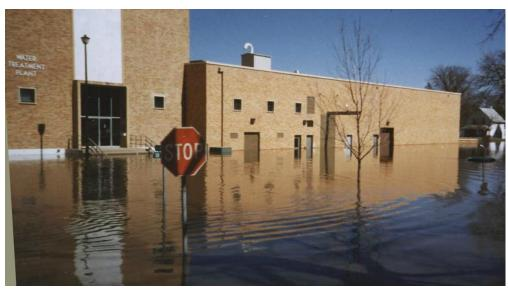
Floodwaters inundated the Grand Forks Water Treatment Plant in April 1997. The city was without drinkable water for 23 days because of the damage to the facility. Photo courtesy of Advanced Engineering, Inc., Grand Forks.
