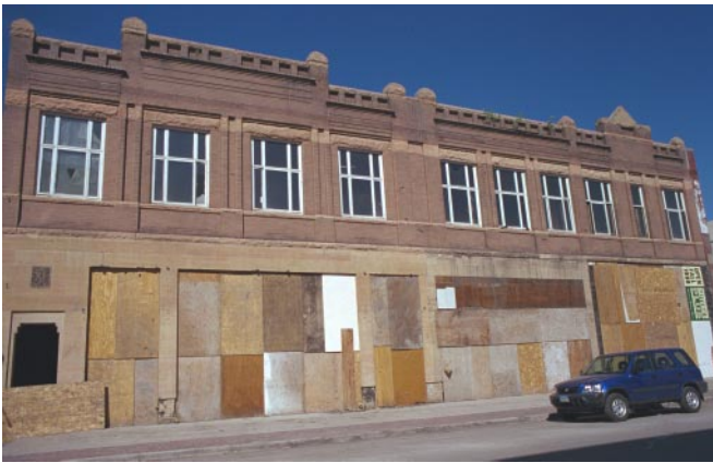
The Phoenix Building in March 2000 as renovation begins.
