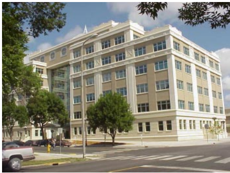
New county office building, completed in January 2000, is better protected from future flooding.
