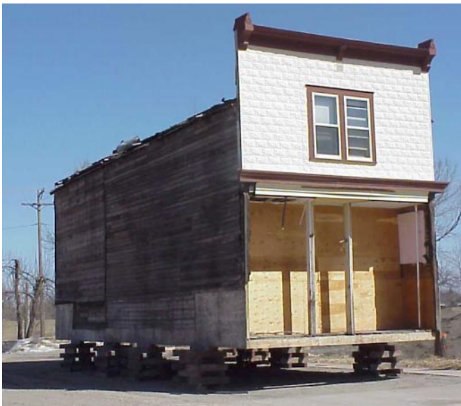
The Boomtown Building, one of Grand Forks’ oldest structures, rests on a pallet base until it can be relocated to the site where it will begin its second century.
