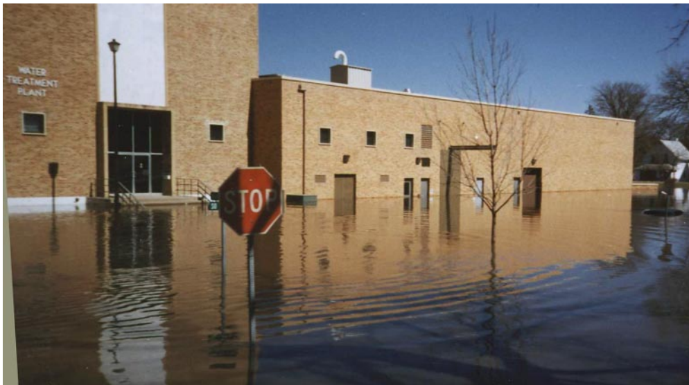
Floodwaters inundated the Grand Forks Water Treatment Plant in April 1997. The city was without drinkable water for 23 days because of the damage to the facility. Photo courtesy of Advanced Engineering, Inc., Grand Forks.
