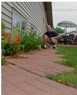
Terry Styf installed pavers with a slight angle to drain water away from his house.
