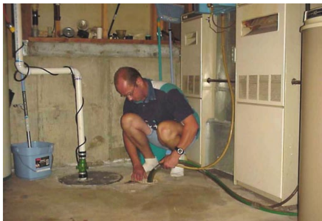
Styf secures hoses into a basement drain.
