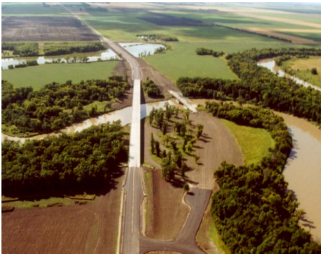
New bridge now provides a safe crossing over the Red River. Photo courtesy of Randy Aarestad, Halstad, Minnesota.
