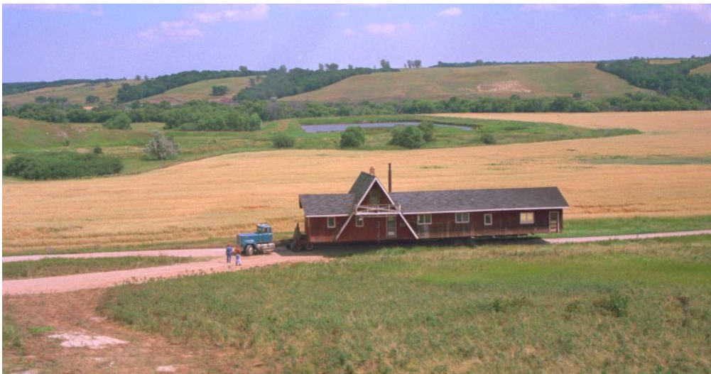
Making the climb... The Scott house is about to ascend to its final resting place overlooking a scenic Barnes County valley. Photo courtesy of Neal Emery.
