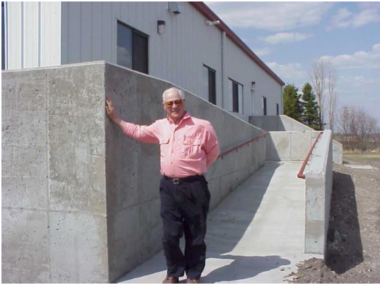
The main floor of the new office and living quarters is 5 feet above the ground level to reduce the chance of flooding again.
