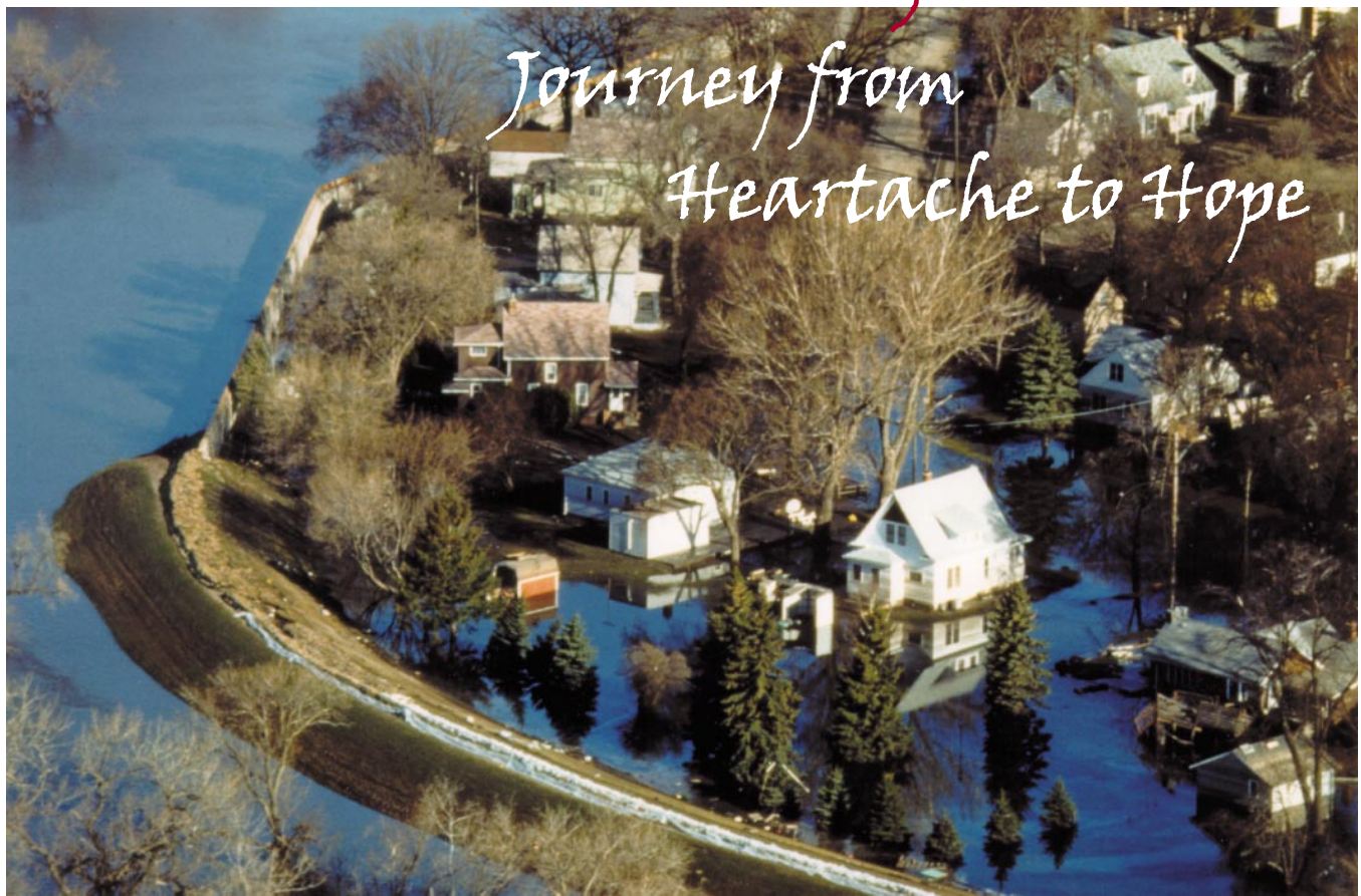
Few neighborhoods in Grand Forks, North Dakota, were spared during the “Flood of the Century” in April 1997. FEMA photo by Andrea Booher.
