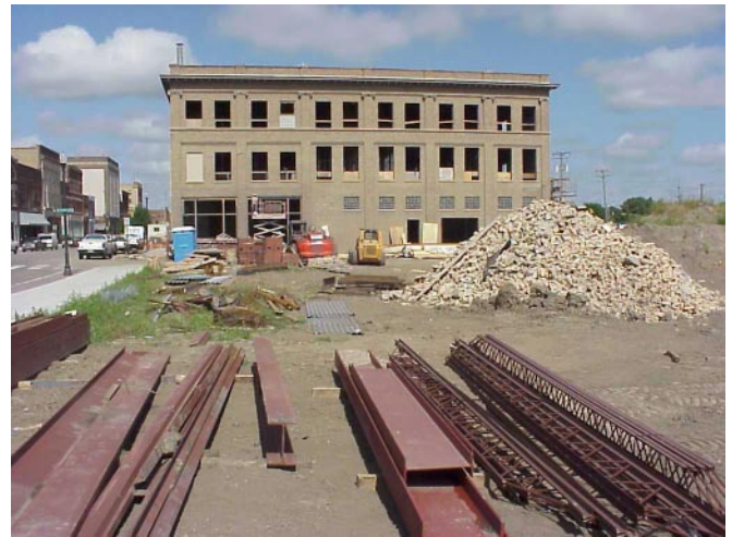
Restoration of the Panovitz Building is well underway.
