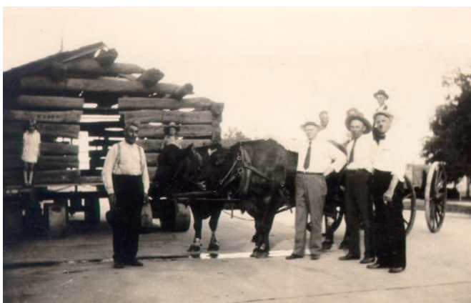
Halvorson's cabin arrives in Hillsboro in 1931. Photo courtesy Traill County Historical Society.
