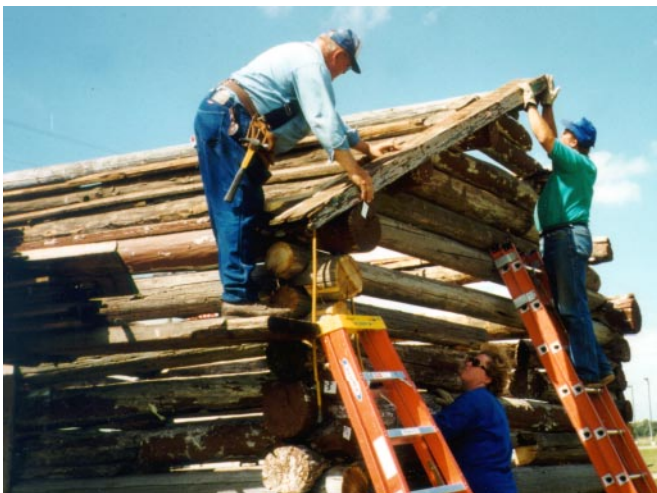
Duane Nysveen (left) gets help taking apart the cabin log by log. Photo courtesy Shirley Nysveen.
