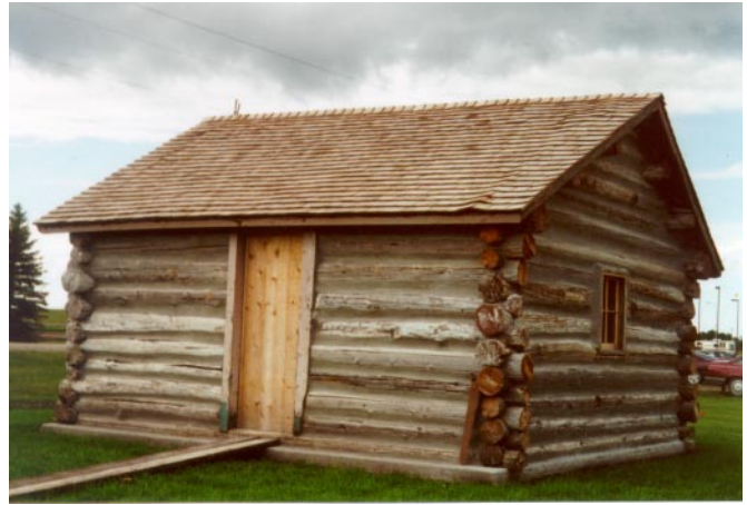
Newly reconstructed outside the floodplain, the cabin now has a chance to live high and dry. Photo courtesy Shirley Nysveen.
