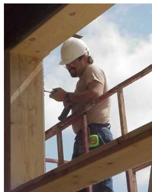
A contractor installs window framing in the Panovitz Building.
