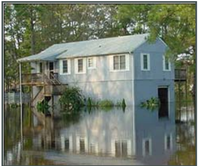
The Stradley elevated residence is out of harms way during flooding caused by Hurricane Isabel.
