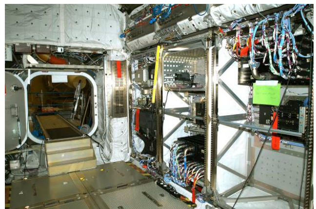
Columbus subsystem racks during testing
