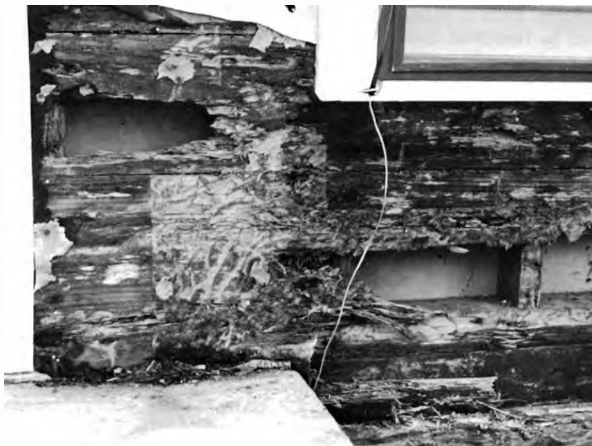
Figure 4. —Termites entered this house from a soil-filled porch.
