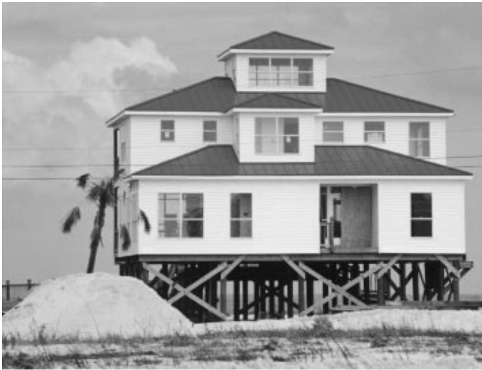
This home was elevated to prevent damage from future storms and flooding. Elevation can reduce flood insurance premiums significantly.
