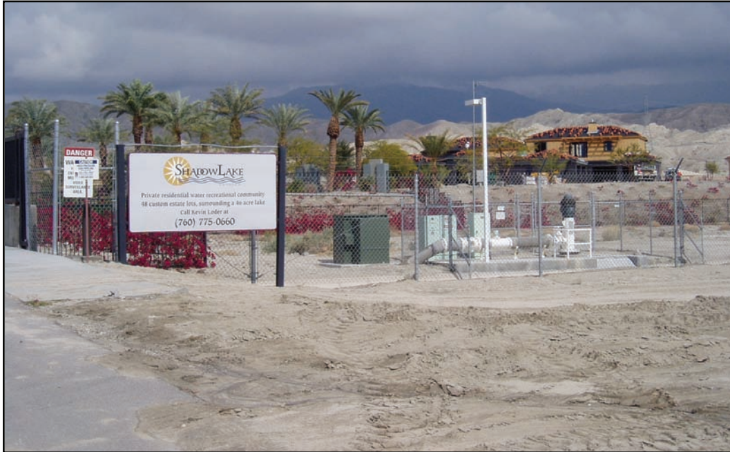
Photograph 5.1 – Shadow Lake gated community/golf course under construction near Indio.
