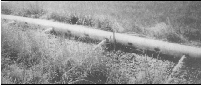
Figure 7-2. Typical Gated Pipe Distribution Unit.
