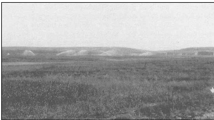
Figure 11-2. Solid set sprinklers apply tomato processing wastewater to overland flow slopes.
