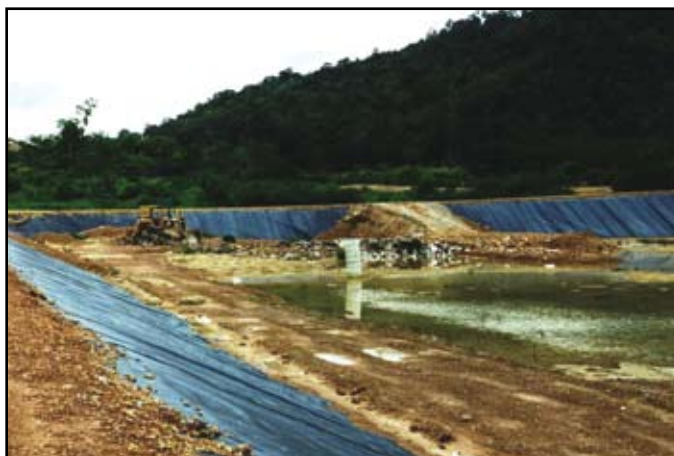
Figure 1-1. A landfill that could pose a risk to local citizens.
