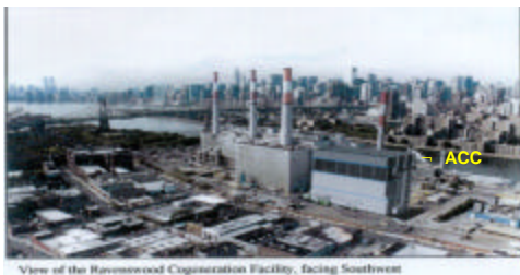
View of the Ravenswood Cogeneration Facility, facing Southwest
