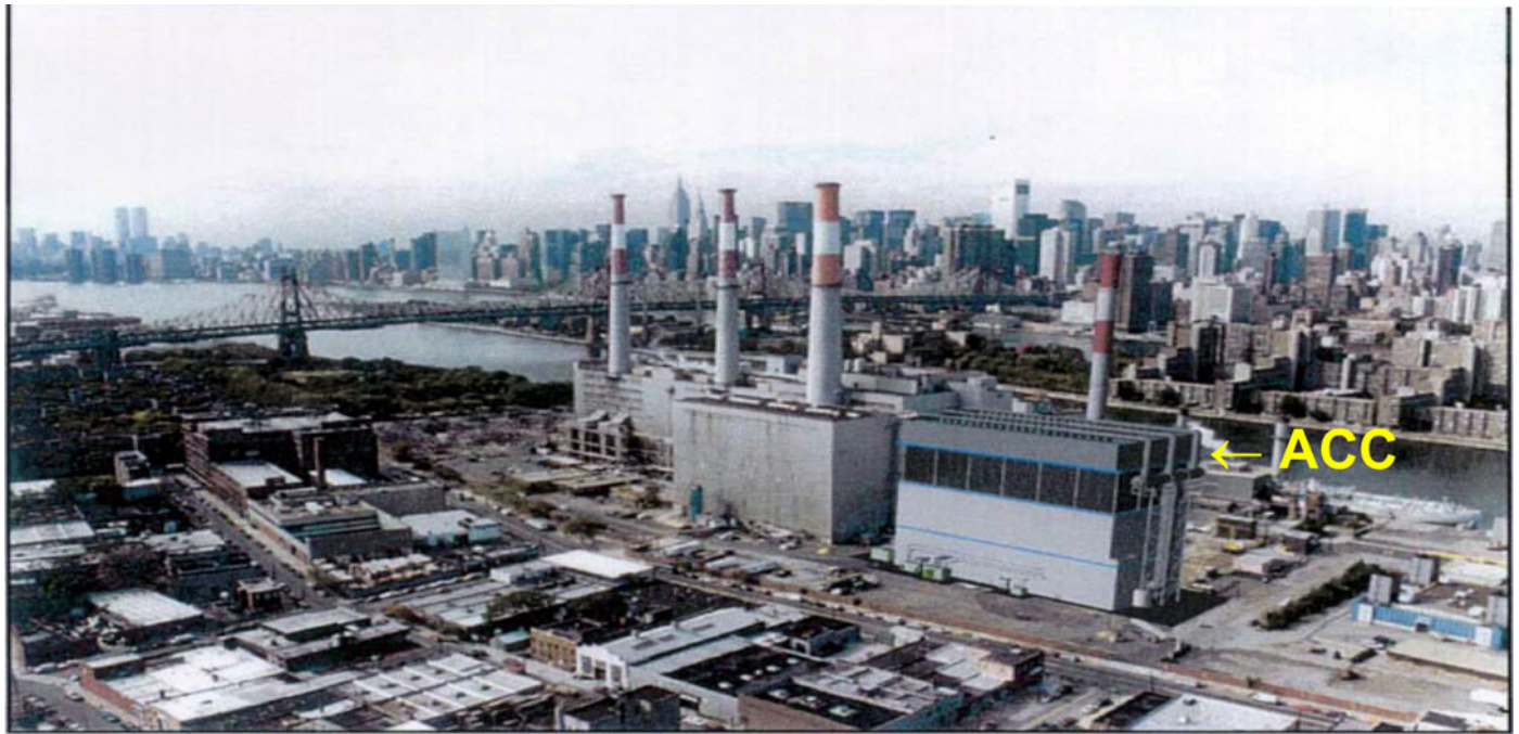
View of the Ravenswood Cogeneration Facility, facing Southwest
