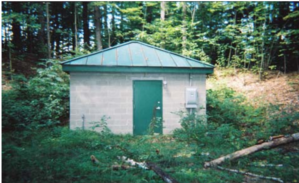
Figure 4-1. Preexisting Treatment Building at Charette Mobile Home Park
