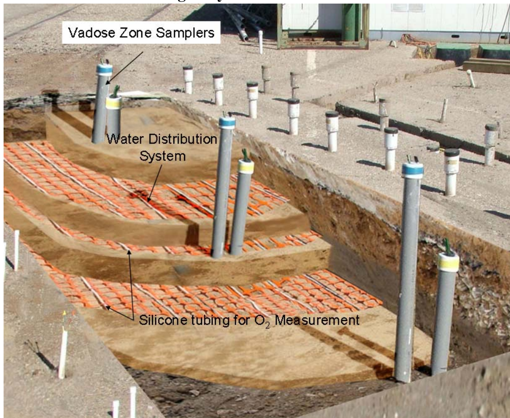
Figure 6. Infiltration gallery as installed.
