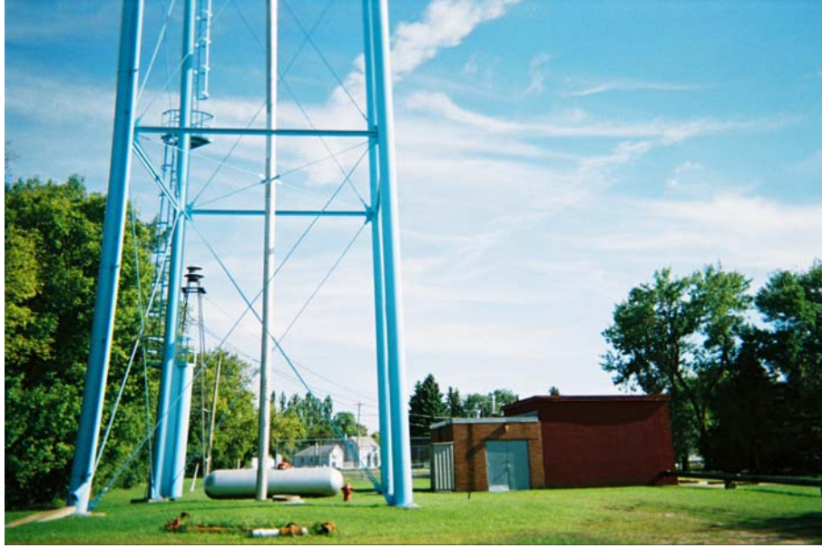
Figure 4-1. Preexisting Pump House at Sabin, MN
