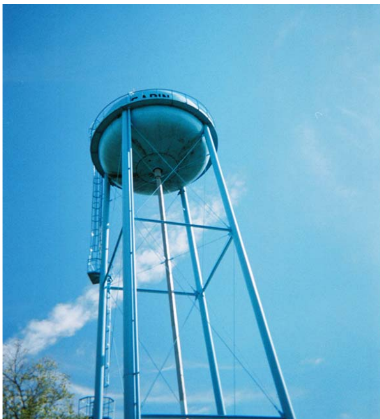
Figure 4-3. Water Tower at Sabin, MN
