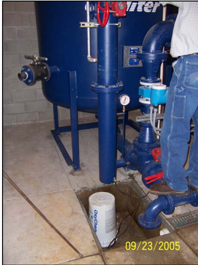
Figure 4-6. Backwash Discharge
