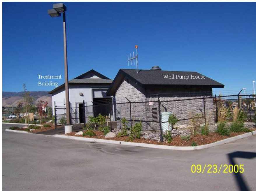
Figure 4-9. New Treatment Building and Preexisting Well Pump House
