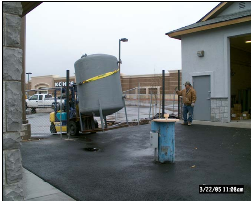
Figure 4-10. Delivery of One Adsorption Vessel
