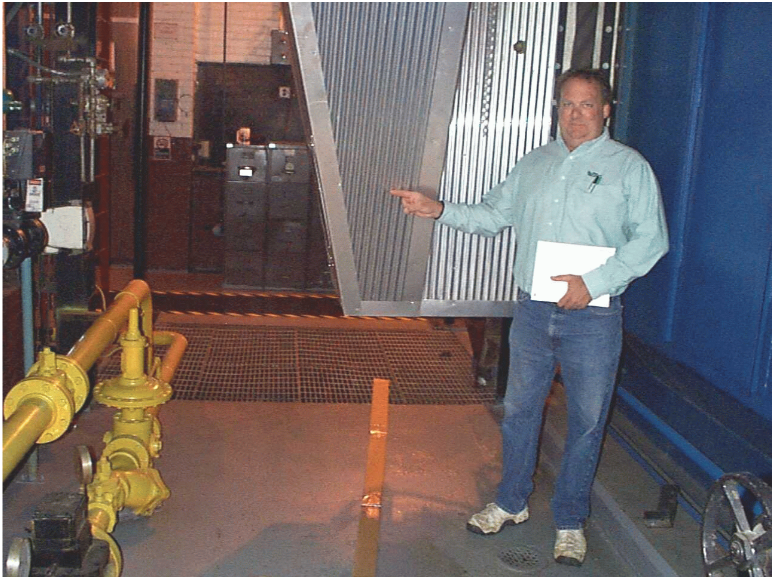
Figure 3-7. Testing area, ground level.
