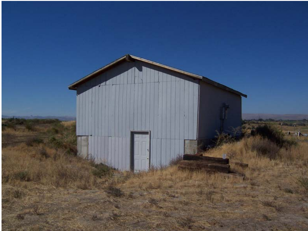
Figure 4-1. Central Pump House at Sunset Ranch Development Site
