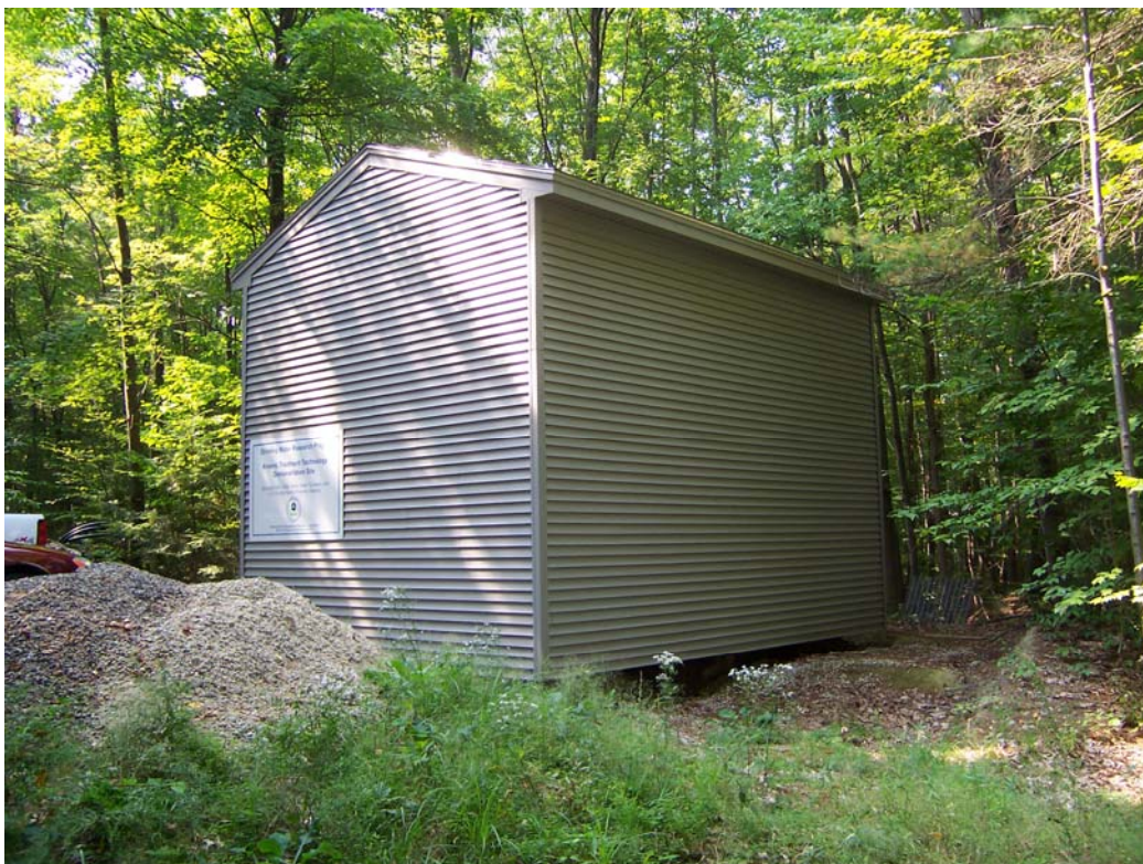
Figure 4-7. New Treatment Building Addition
