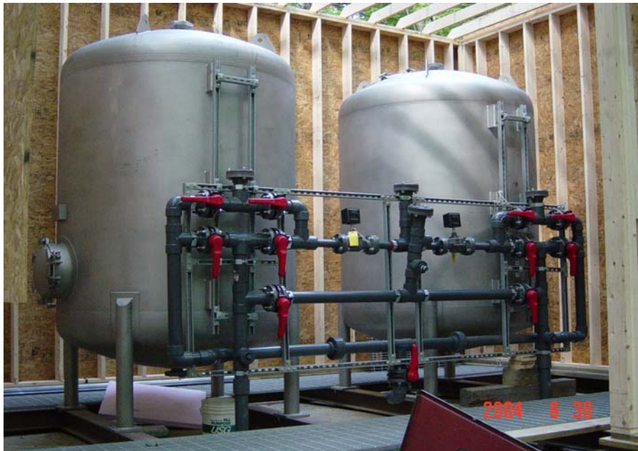
Figure 4-6. ADI G2 Media Arsenic Adsorption System
