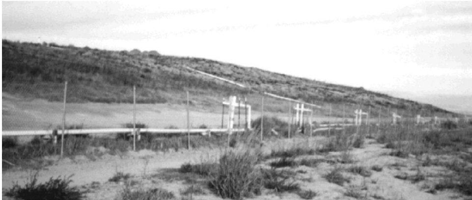
Figure 3-5. Abandoned Horizontal Barrier Trench System.
