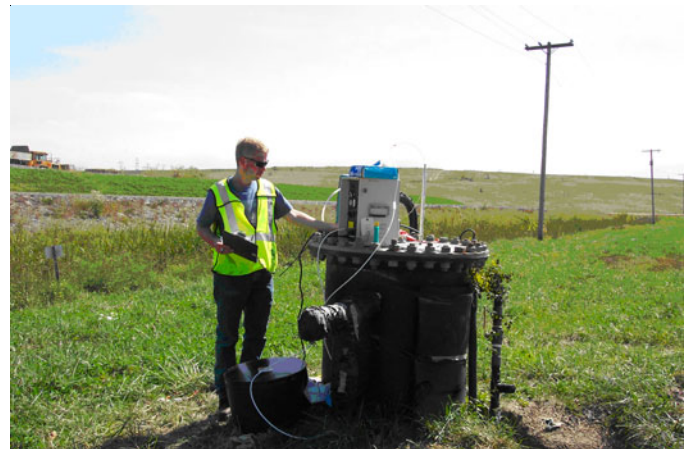
Figure 50. Mercury Sampling Conducted at a Landfill Gas Header Access Point Located Upstream of the Main Flare Station.
