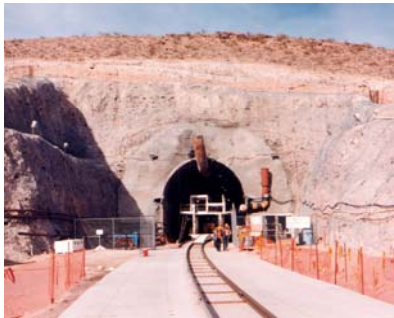
Figure 2 - Yucca Mountain Entrance Tunnel
