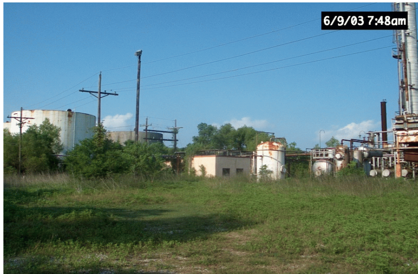
East Facility process area - Before
