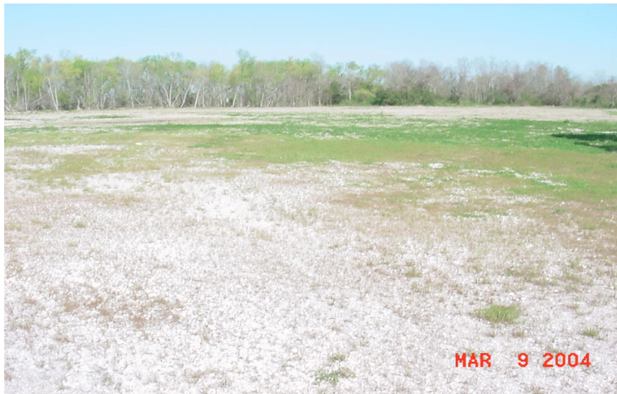
West Facility - After
