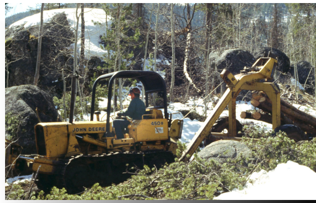
Figure 9. Thinning and removal of beetle infested trees and hazard trees.
