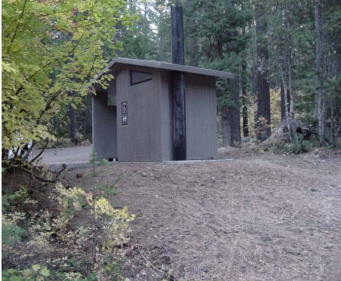
Low maintenance toilet facilities, designed to blend with a Forest setting, were selected to enhance visitor experiences in campgrounds.
