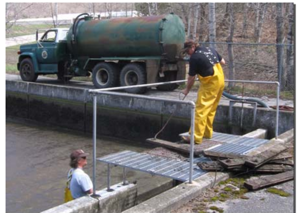
Maintenance Mechanic Bob Petersen and Fisheries Biologist John Johnston cleaning the settling basins. - Photo by Clarice Beckner
