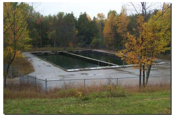
Off-Line Settling Basins
