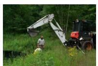
The Six-Tile water supply is dredged and pumped out annually to reduce the accumulation of bacteria-laden sediment, and thereby, reduce the risk of disease. It typically takes one to three days depending upon the amount of debris. The area above the head dam is first dredged with the use of the Bobcat and bucket attachment. Then Bob Petersen dons his wet suit and
