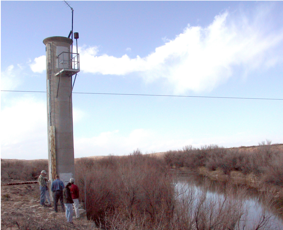
Red Bluff Gauge near New Mexico-Texas state line
