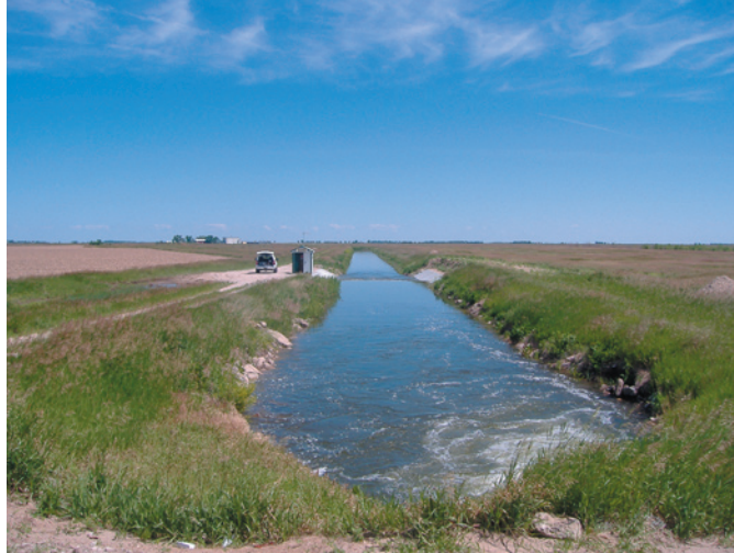
The recently installed long-throated flume in the Airport Lateral at Ainsworth Irrigation District. A solar-charged radio/control unit is housed in the building at left of the flume.
