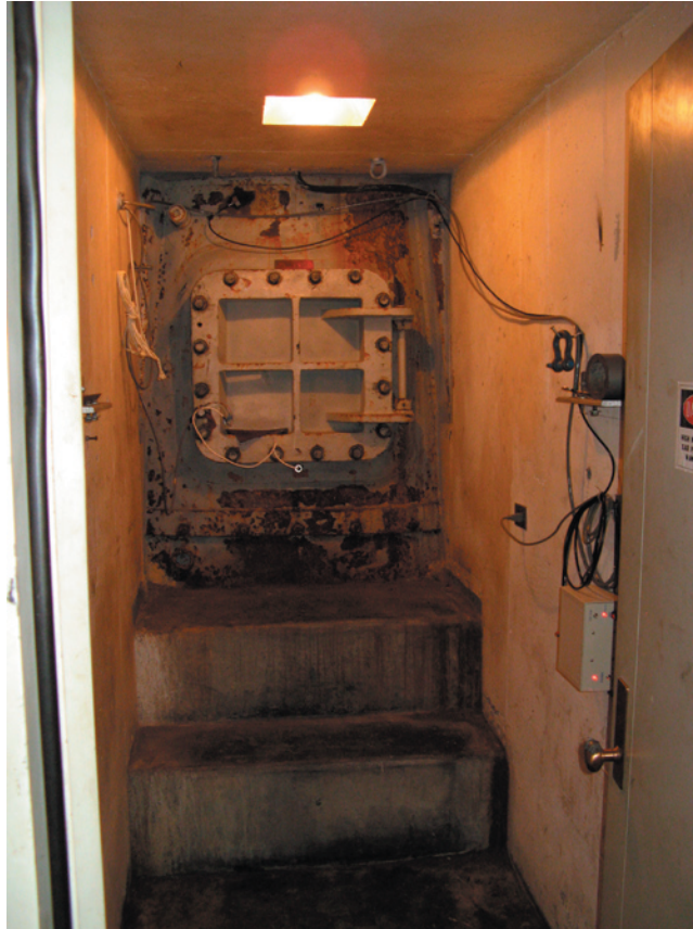
Cavitation system detection installation.
