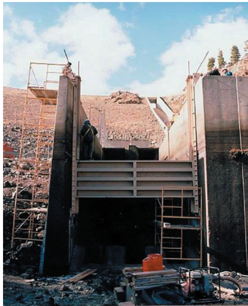
Flow deflector during installation at Mason Dam in October 2002.
