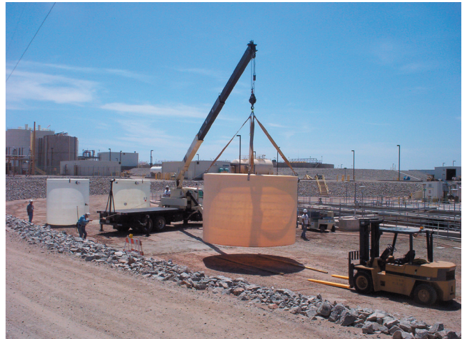
Positioning of tanks to contain pilot slowsand filters at the YDP (July 2004).
