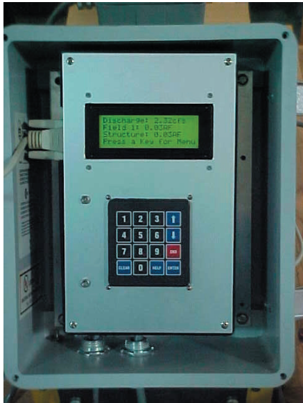
Upgraded CFM unit installed on the WRRL canal model
