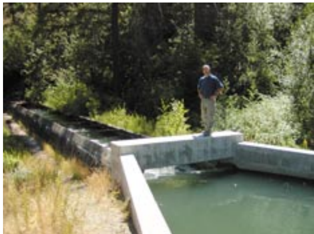
Tieton Diversion Canal with 235-cfs flow.
