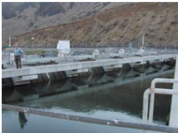
The Rosa Diversion Dam fish screens on the Yakima River north of Yakima, WA .
