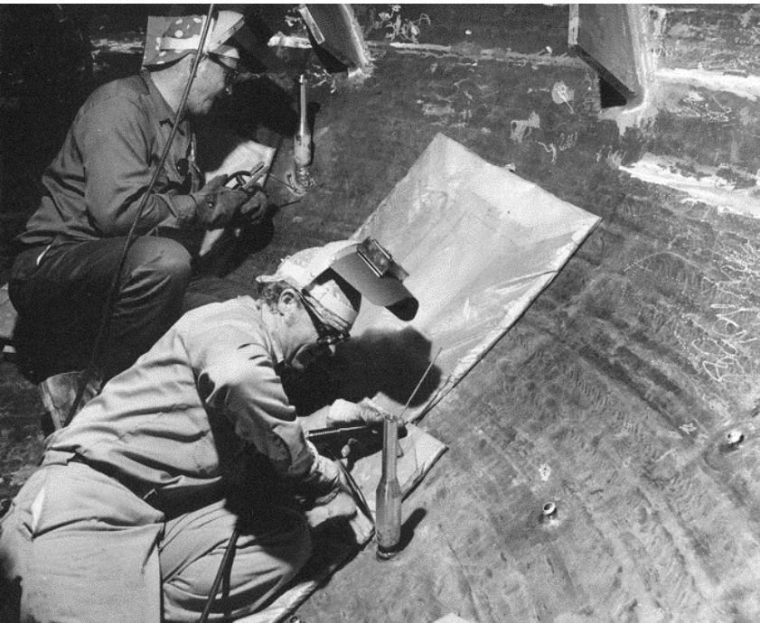
Repair in Process
