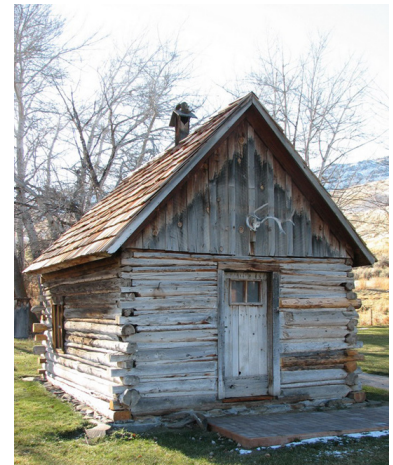
The log house is now more structurally sound.
