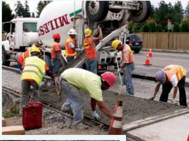
Roads Division trial of porous concrete sidewalks
