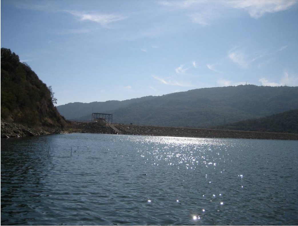
Figure 3.7-1a. Casitas Dam and Spillway
