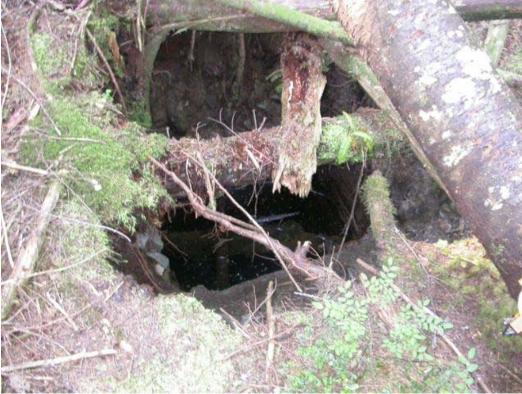
Photo 5. Close-up of flooded shaft collar which poses a serious physical hazard at the Site (photo by G. Graham, 6/22/2004).
