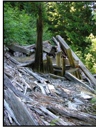
Photo 12. Crusher Base, July 2006
