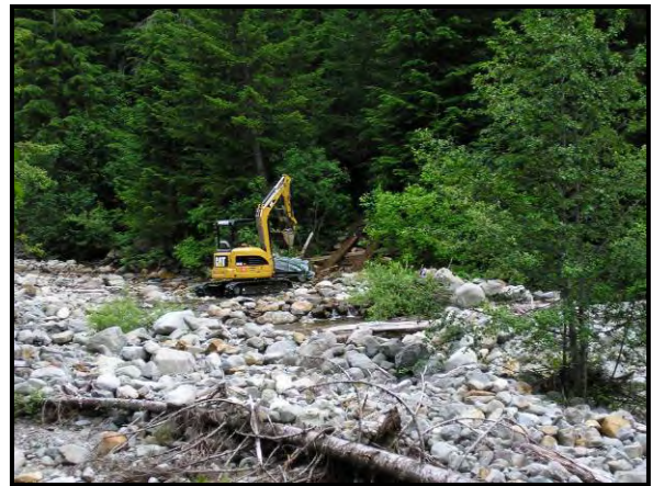
Photo 6. Abandoned access Road, July 2006
