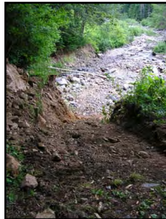
Photo 38. Excavator Access Ramp, July 2006
