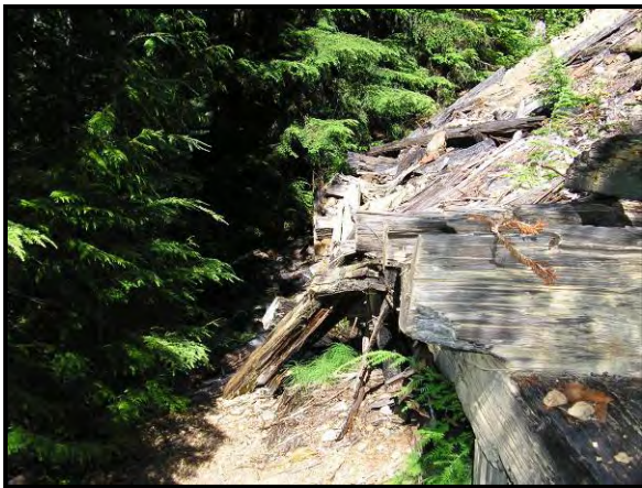
Photo 11. Ore Bin Railway, July 2006
