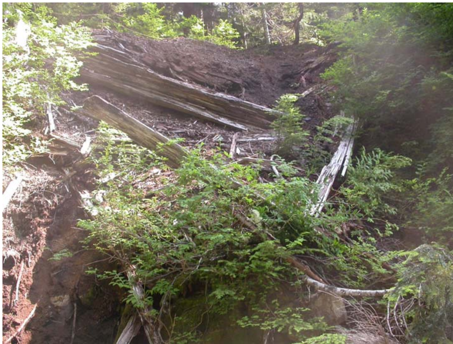
Photo 4. Sidney Mine waste rock dump as viewed from 76 Creek looking towards Photo 3. Note slumping of material as a result of 76 Creek eroding into the toe of the dump, view to the northeast (photo by G. Graham, 8/3/2006).
