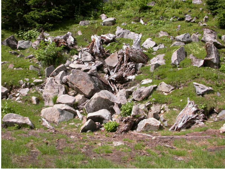
Photo 3. Collapsed portal of Pride of the Woods Mine adit, no mine discharge or evidence of mine discharge was observed, view to the west (photo by G. Graham, 8/2/2006).
