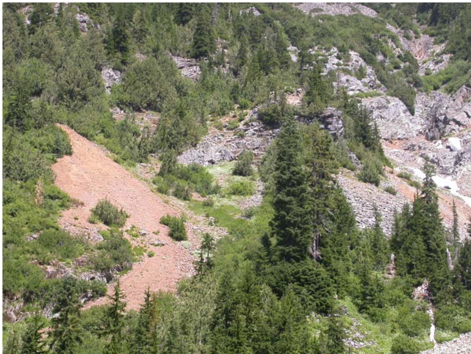
Photo 10. Pride of Mountains Mine as viewed from Glacier Basin, view to the northeast (photo by G. Graham, 8/2/2006).
