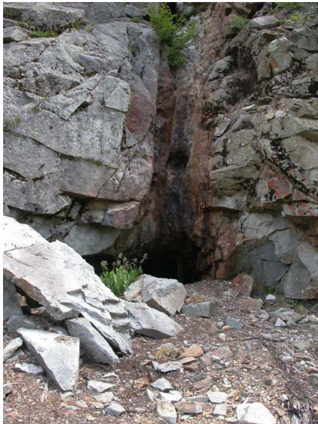
Photo 6. Portal of northwest adit at the New Discovery Mine. No mine drainage or evidence of mine drainage was observed, view to the east (photo by G. Graham, 8/2/2006).
