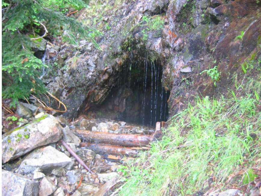
Photograph 7. View east at the Reservoir Adit. (CES 6-29-05)
