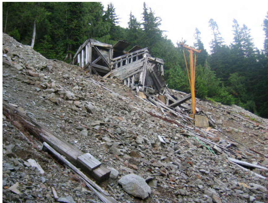
Photograph 12. View southeast at the upper tram terminal and waste rock at the Kromona Mine. (CES 6-29-05)
