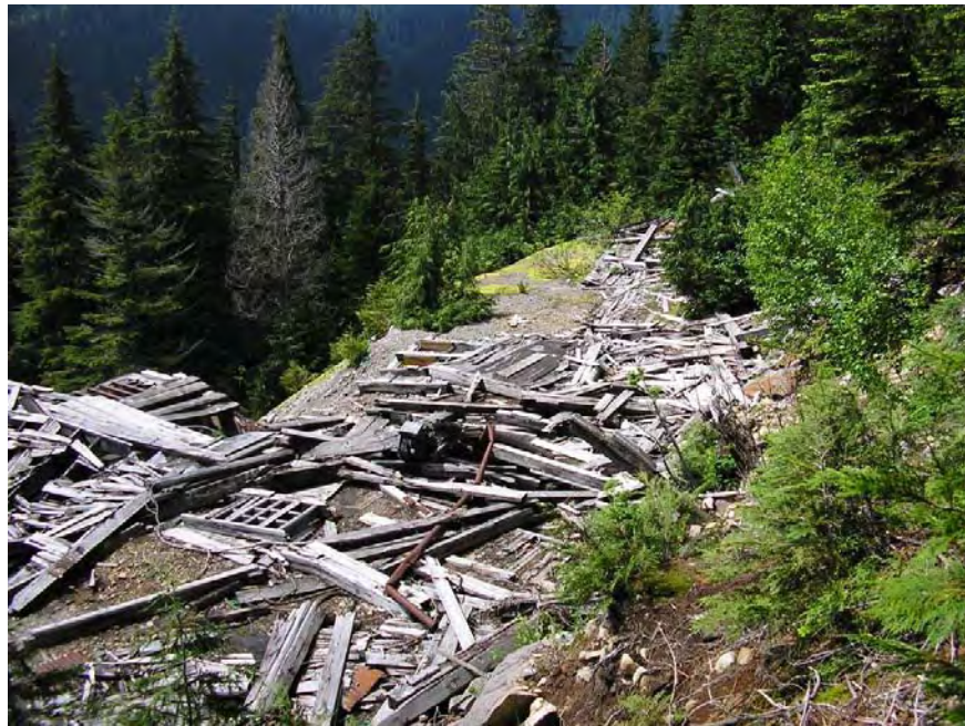
Photograph 10. View north at debris at upper (Main Adit) level at Kromona Mine. (CES 6-28-05)
