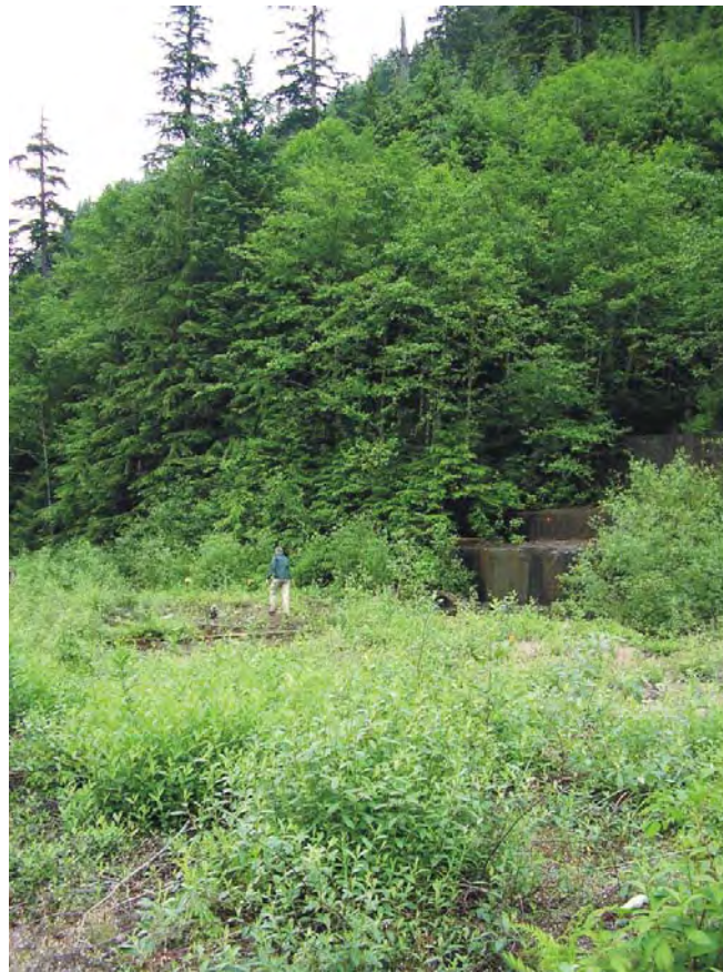
Photograph 14. View east at Kromona Mill foundation and tailings area. (CES 6-29-05)
