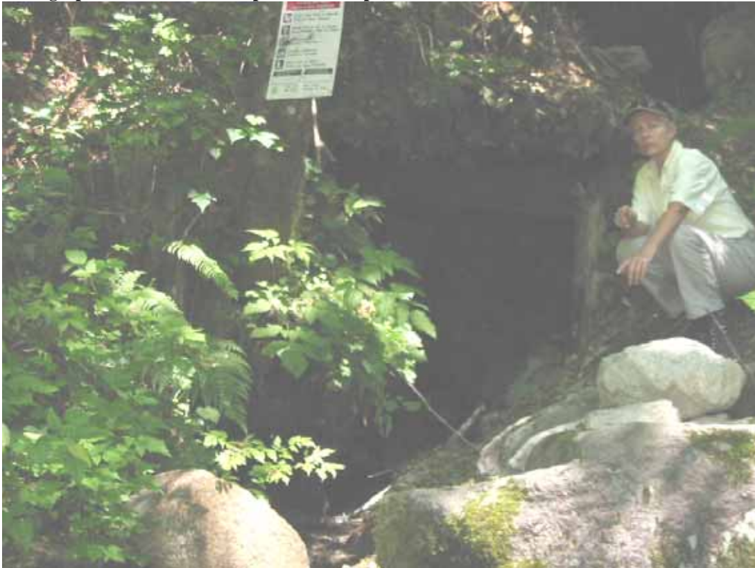
Photograph 12: Closeup of Adit 2 Portal (CES 6-22-04)
