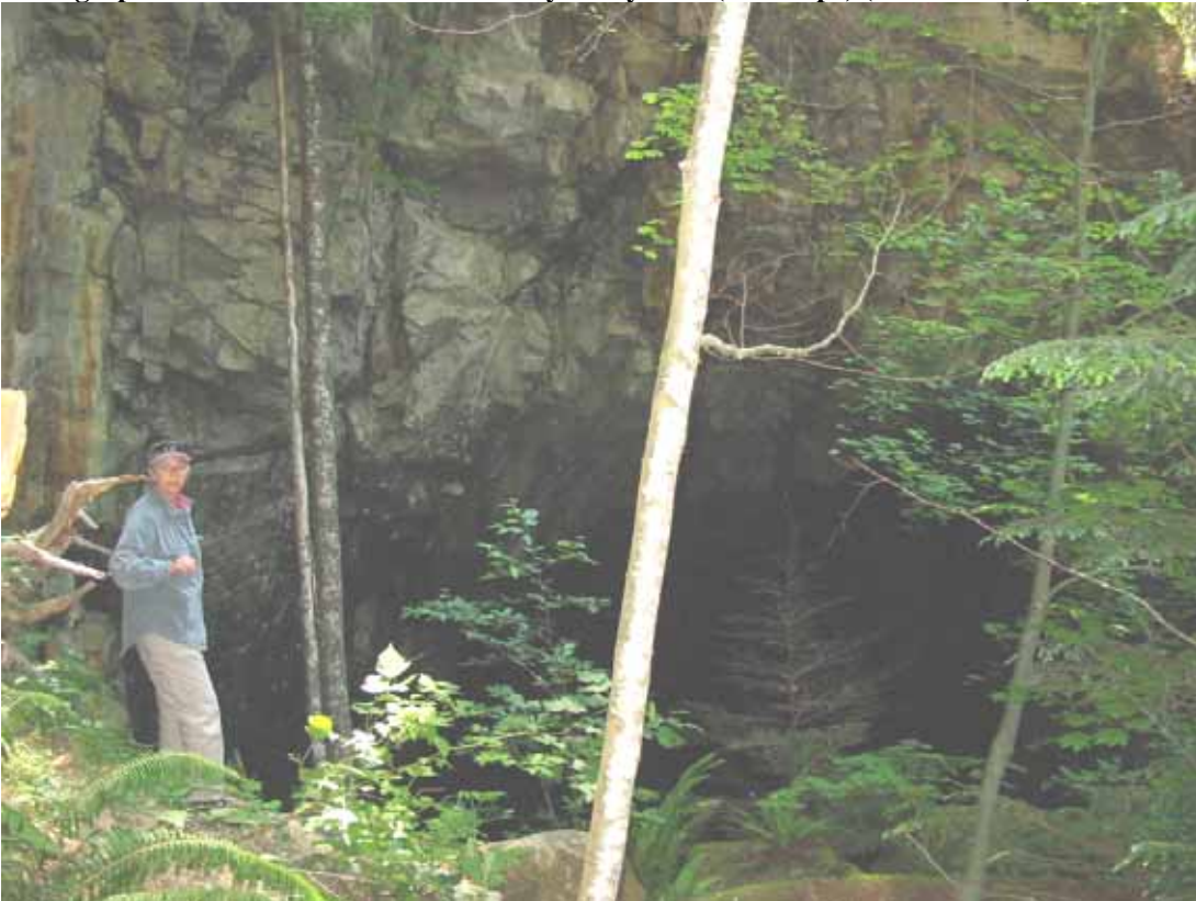
Photograph 16: View southeast at the caved west stope above Adit 3 (CES 6/22/04)
