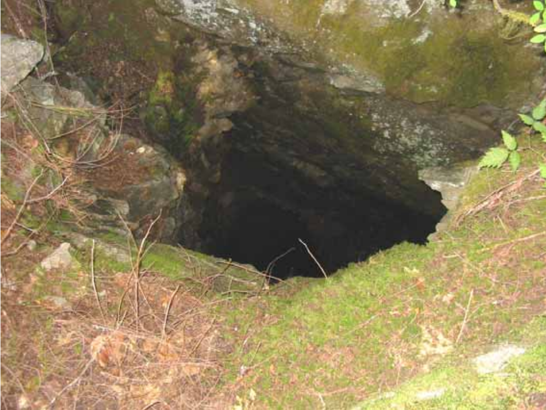
Photograph 17 View north at the ventilation rise above Adit 3 (CES 6/22/04)
