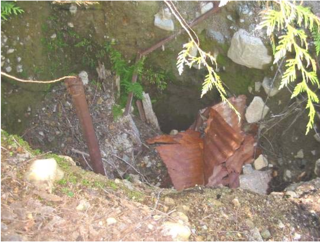
Photograph 19: Looking down into shaft at Rainy Mine. CES 6/27/04
