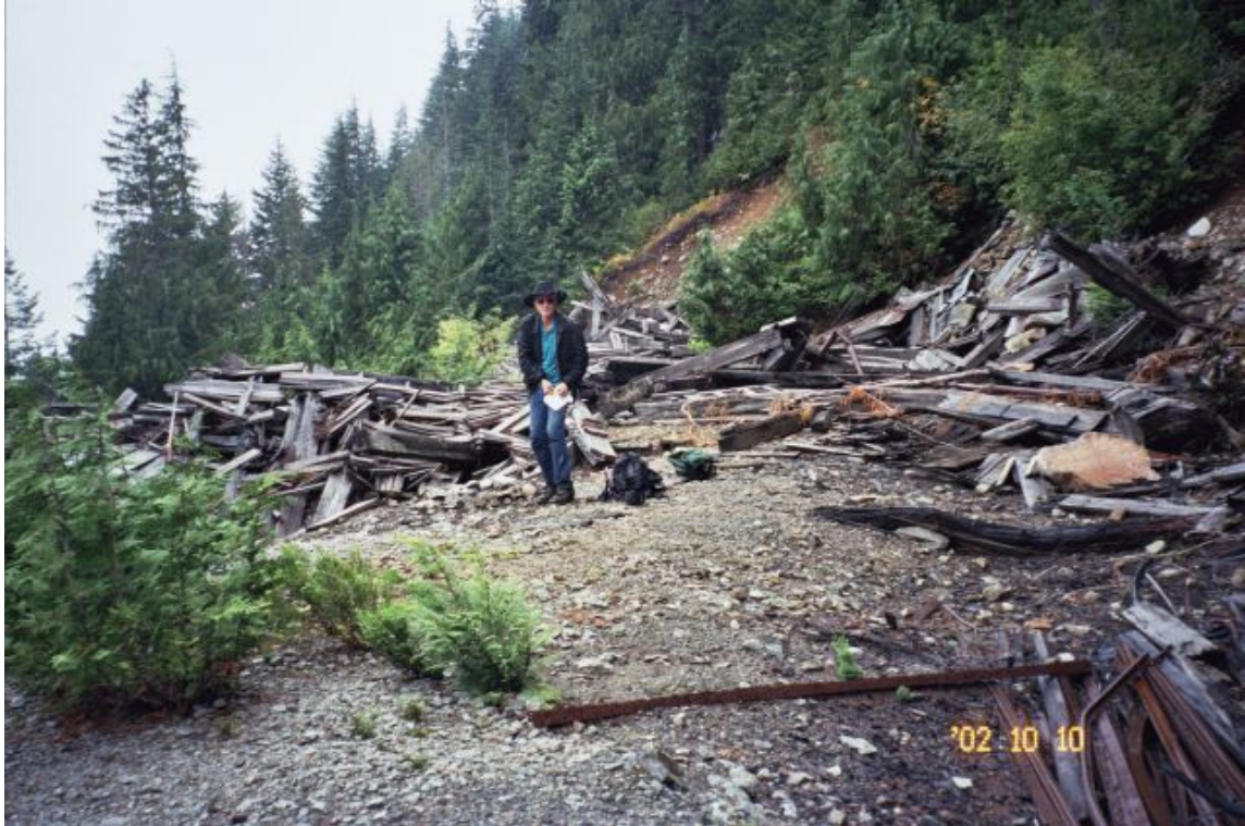
Photo 5. Refuse atop waste dump at main adit/upper tramway terminal where bunkhouse, cookhouse, and workshop were located, view to the northwest (photo by G. Graham, 10/10/2002).
