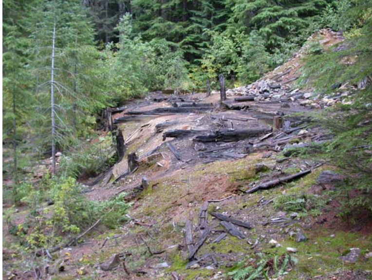
Side View of The Concentrator Foundation
