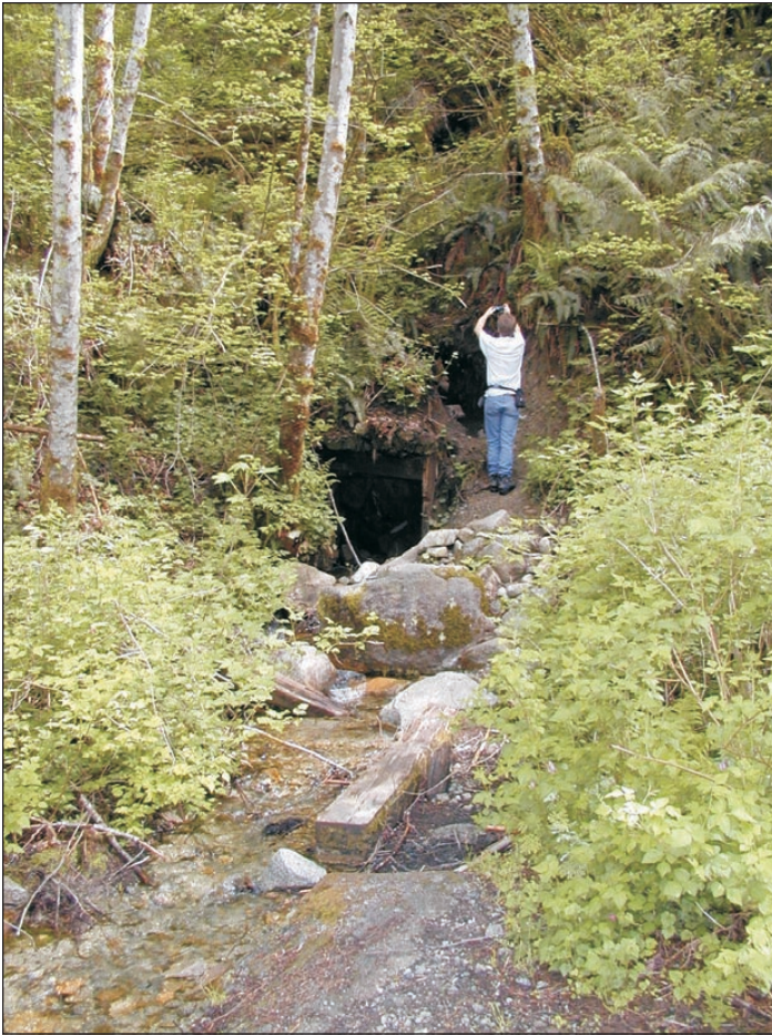
Figure 7. (above left) Main haulage level, adit 2. The tunnel is caved beyond the DGER geologist. A discharge stream is in the foreground.
