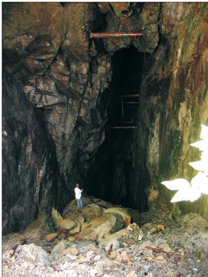
Figure 11. Entrance to stope 11 on vein centerline. Note the 1-foot-diameter stulls overhead. The back of the stope is 220 feet distant. View is to the east.
