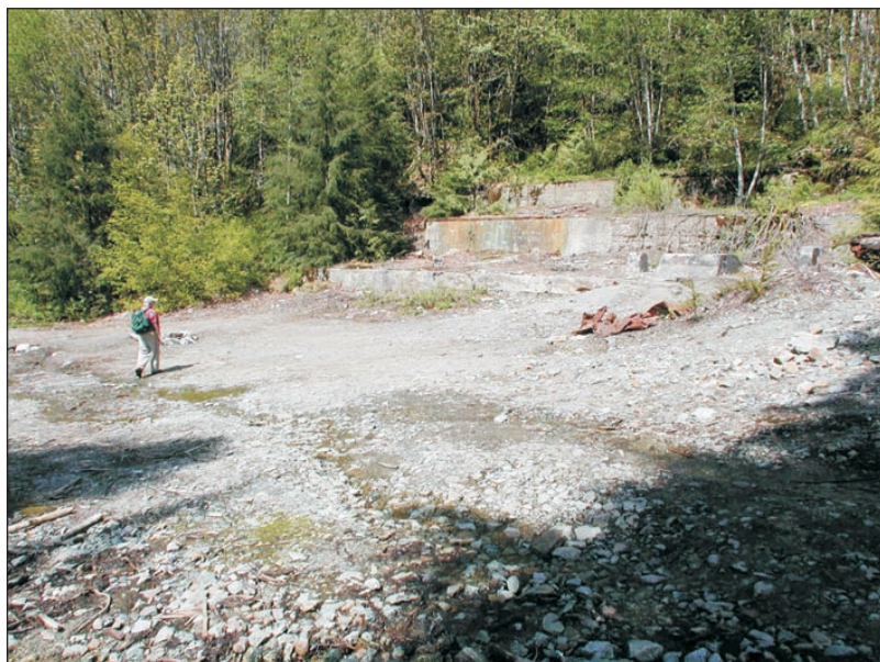
Figure 14. Mill foundation. Former waste-rock site in foreground was washed away during Trout Creek flooding. Note machine gun bullet holes in foundation.
