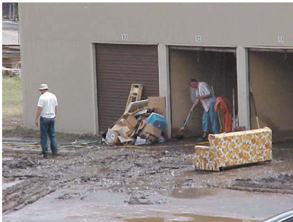
Figure 2. Flooding aftermath from the storm of May 27, 2001, in a storage building constructed in the poorly defined Cave Gulch stream channel, near Helena, Montana.
