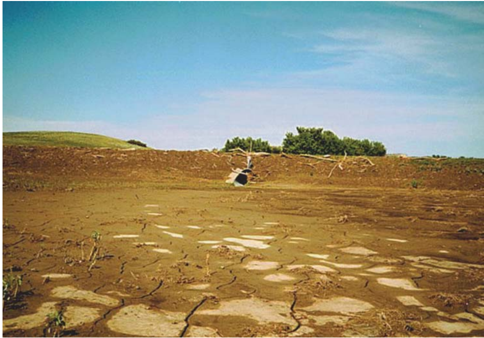
Figure 4. Sediment-laden floodwaters on Brian Creek near Ashland, Montana, overtopped the road and deposited a thick layer of muddy sediment (foreground) and large, woody debris (road embankment in background). Note the person standing on the culvert for scale. View is looking downstream.
