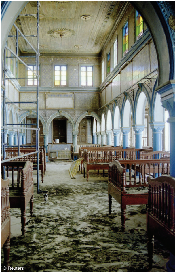
Bomb damage to a Jewish synagogue in Djerba, Tunisia, after terrorists exploded a tanker truck containing cooking gas outside the synagogue, killing 17 persons, 11 April 2002.
